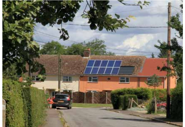
Solar panels, Grove Park Rita Gardner © RGS-IBG Discovering Britain
