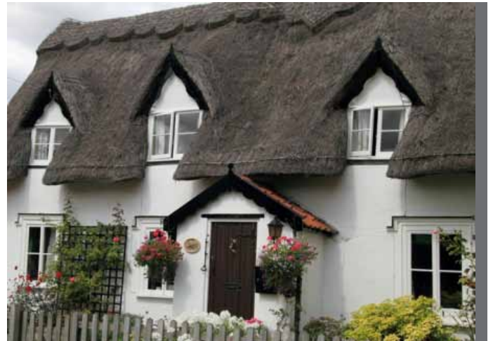
The White House with its wheat thatch roof Rita Gardner © RGS-IBG Discovering Britain
