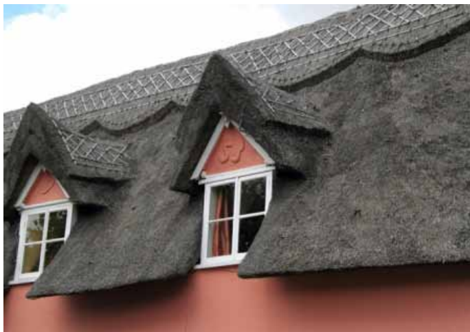
Willow Cottage's water reed thatch roof Rita Gardner © RGS-IBG Discovering Britain
