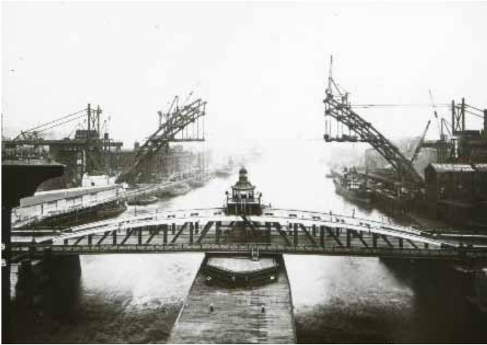
The Tyne Bridge under construction, 1928 Wikimedia Commons (Creative Commons License)
