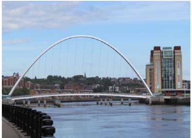
Gateshead Millennium Bridge and BALTIC Centre Rory Walsh © RGS-IBG Discovering Britain
