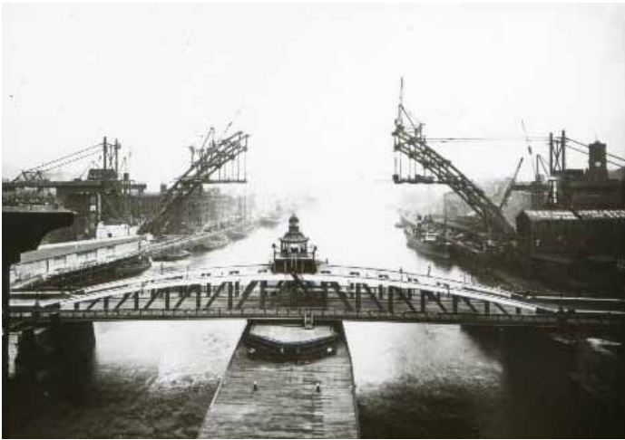
The Tyne Bridge under construction (1928) Wikimedia Commons (CCL)
