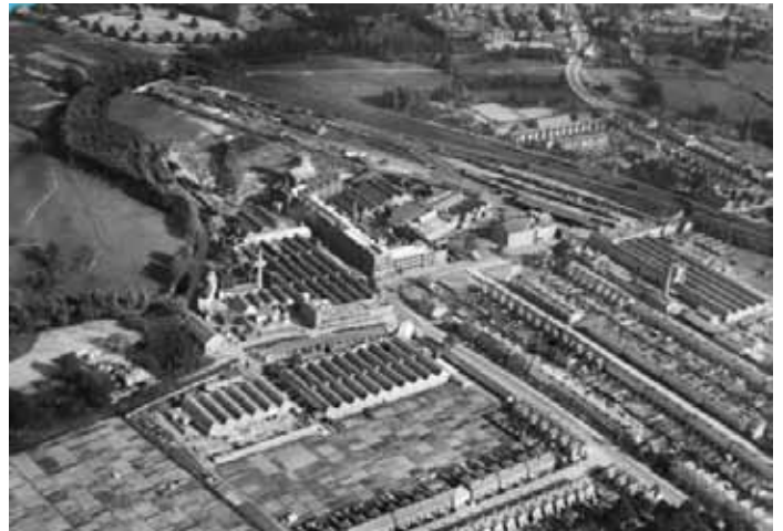
Industrialised Chelmsford Courtesy of www.britainfromabove.org.uk © English Heritage
