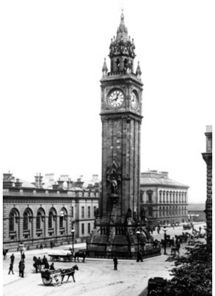
Albert Memorial Clock, 1897 - already leaning over to the side where it was built on the banks over the River Farset Wikimedia Commons
