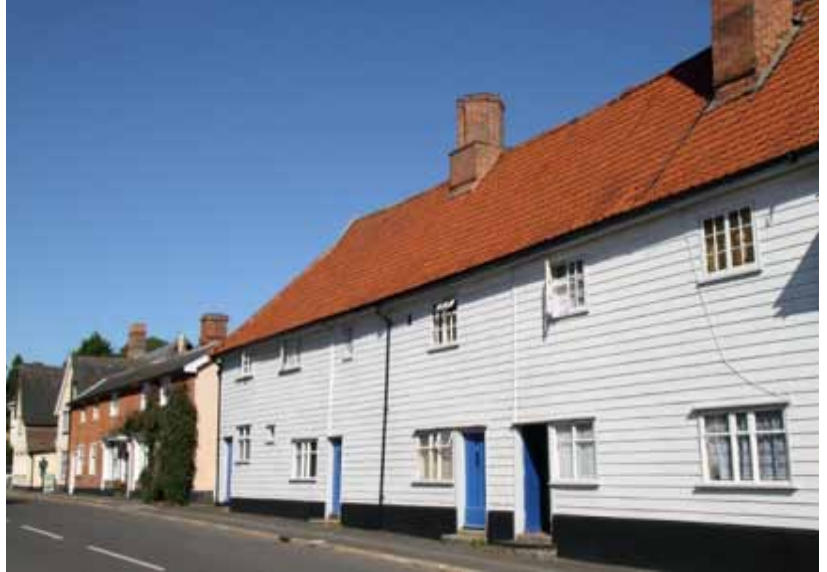
The former Guildhall © Rita Gardner
