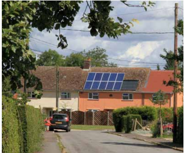
Solar panels, Grove Park © Rita Gardner
