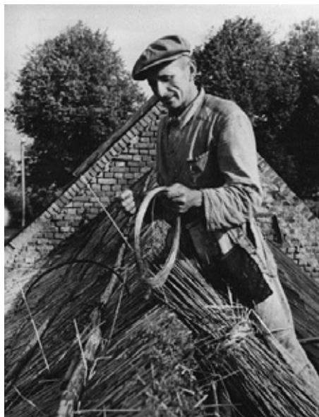
A thatcher building a straw roof (1949) Wikimedia Commons (CCL)
