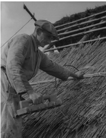
A thatcher building a straw roof (1949) Wikimedia Commons (CCL)
