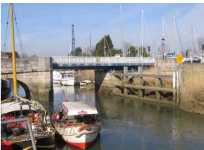
The town bridge, rebuilt using funds raised by the tolls Rory Walsh © RGS-IBG Discovering Britain
