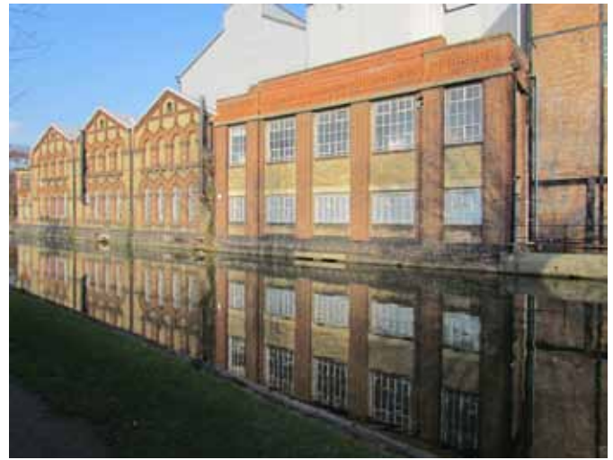
The building that electrified Oxford Rory Walsh © RGS-IBG Discovering Britain
