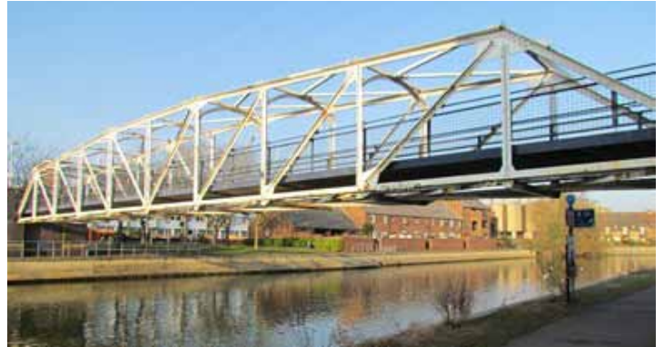
Gasworks pipe bridge Rory Walsh © RGS-IBG Discovering Britain
