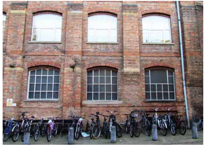
Hyde's functional factory building Rory Walsh © RGS-IBG Discovering Britain
