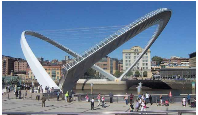
Gateshead Millennium Bridge when open © Mike1024, Wikimedia Commons (CCL)
