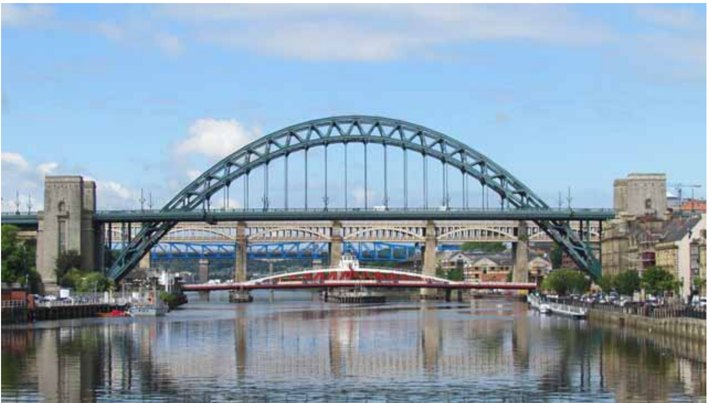
The view of the older Tyne bridges from Gateshead Millennium Bridge © Rory Walsh
