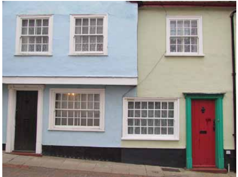
The large ground floor windows of the weavers' cottages Rory Walsh © RGS-IBG Discovering Britain
