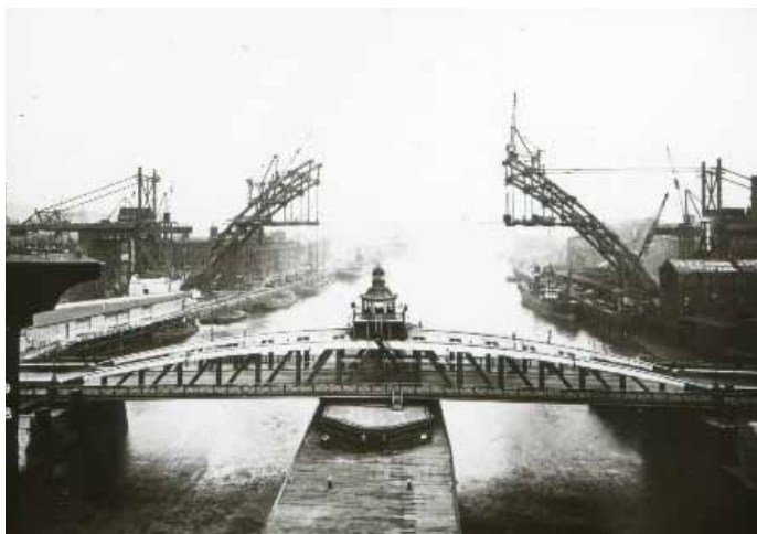
The Tyne Bridge under construction, 1928 Wikimedia Commons
